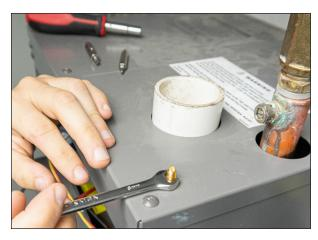
Use a 8mm wrench to remove the antenna connection.
