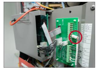
Remove the SRC boiler cable from the Outdoor sensor terminals (7, 8).
