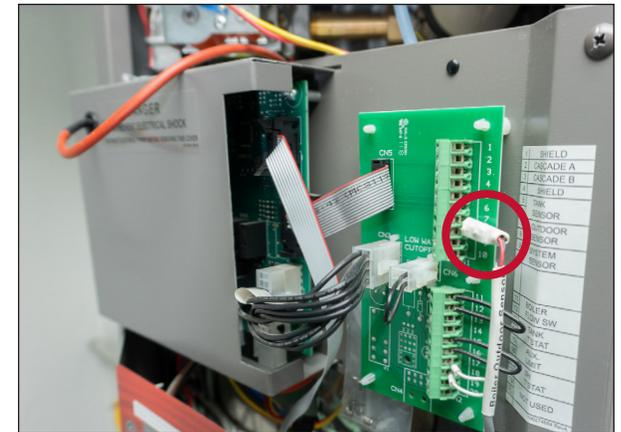
Remove the SRC boiler cable from the Outdoor sensor terminals (7, 8).
