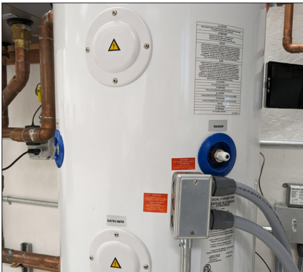
Buffer Tank with Boost Heat
