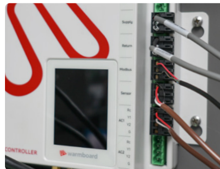
Modbus terminal wired (Red, Black, Ground)
