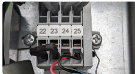
SIM Modbus spring terminal bar.
