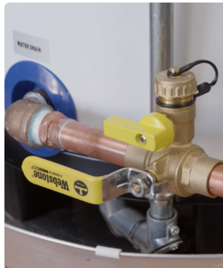
Drain ball valve and glycol feeder line
