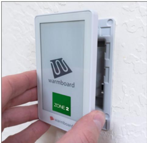
Thermostats should be installed after texture and paint. Each thermostat snaps into a pre-wired J-Box (at least 18 cu. inches). Once the Warmboard thermostats are powered up, they communicate wirelessly, so no additional wiring is required.
