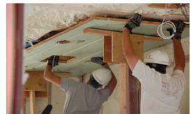
Warmboard Installation of Ceiling Panels at Refract House
