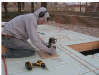
Warmboard Installation at Ohio State's "Ohio-centric" House
